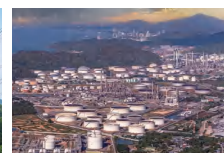
Oil & Gas Infrastructure Inspection
